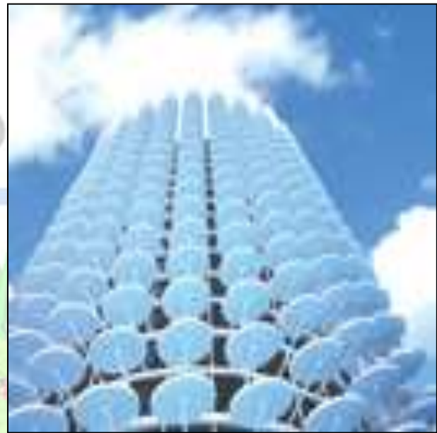
Figure 2: Installation of Solar Panels around the periphery cooling towers
